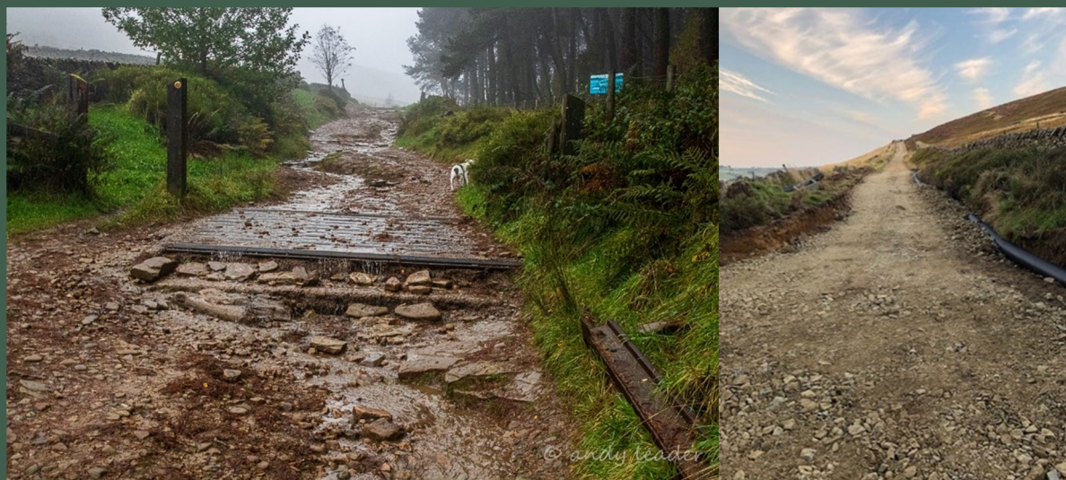
Image 3 | Ramsden Road before and after PNFS intervention
