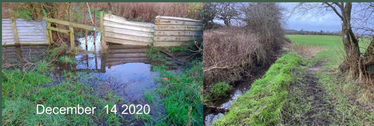
Image 9 | Stockport path 119 before and after PNFS intervention
