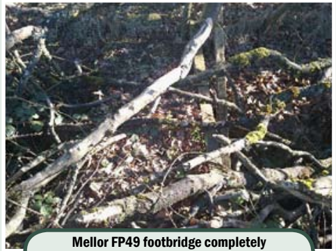
Mellor FP49 footbridge completely covered by tree branches
