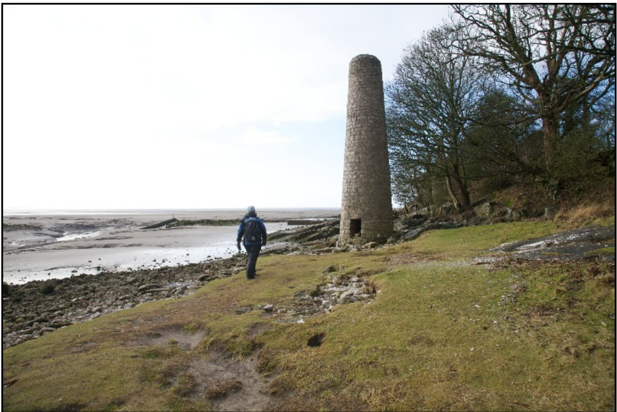
Beyond the chimney lies the 'Rocky Foreshore' opposite
